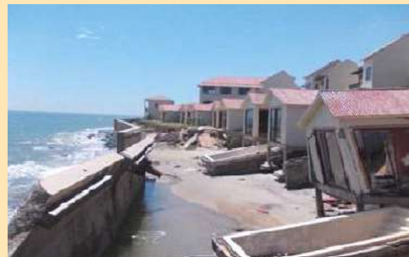
Hotels in Cua Dai (Hoi An) damaged by coastal erosion.
